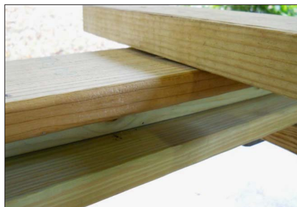
Figure 3. The channel for dropping the plywood gate is formed by fastening a smaller board between two larger boards. Photo by Becky McPeake, University of Arkansas.
