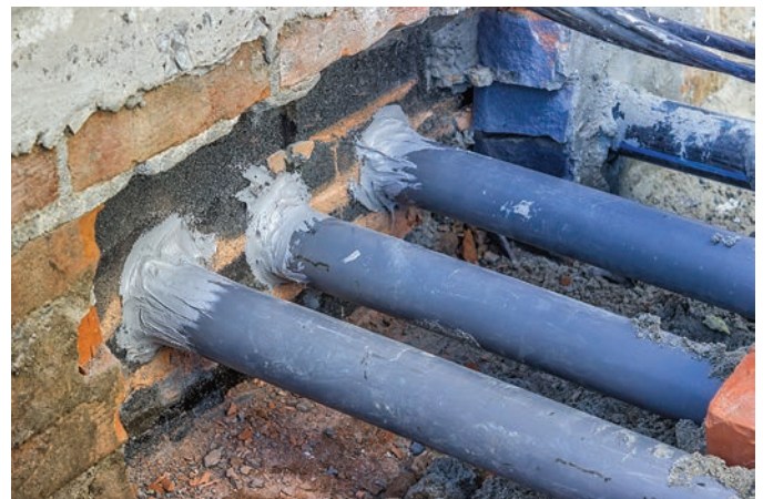
Figure 5. Seal holes with rodent-proof materials where pipes, wires, or similar objects enter buildings.
